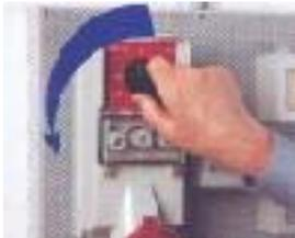
Cut off power to the line switch and disconnect the equipment power cable.
